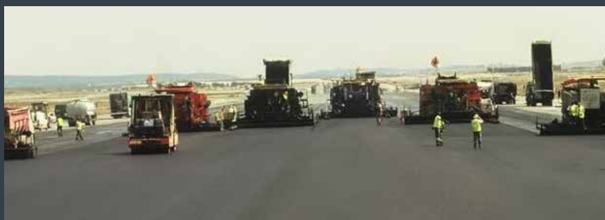
Echelon paving the main runway on the Charles De Gaulle airport in Paris.
