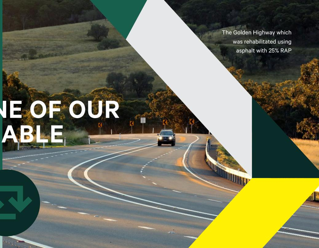
Asphalt is 100% reusable which means that at the end of its service life it can be reused to produce new asphalt. Reclaimed Asphalt Pavement should not be considered as a waste but an engineered product. Therefore RAP should not be disposed of but reused in the production of new asphalt.
